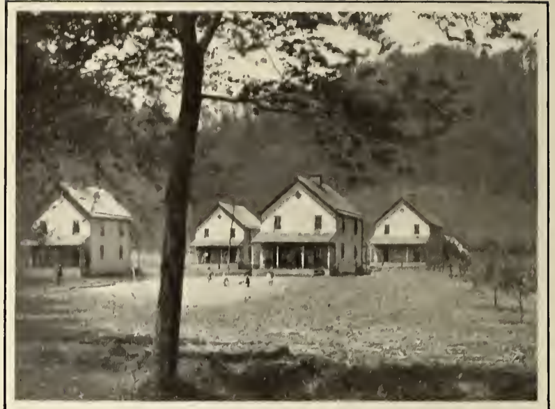
These are some of the cottages which have been erected by the students in order to pay their room-rent
